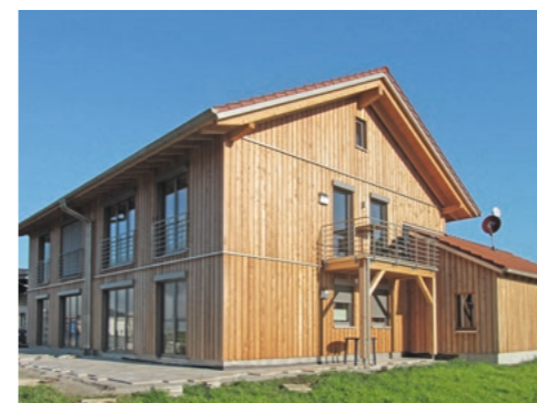
Semi-detached house in timber construction
