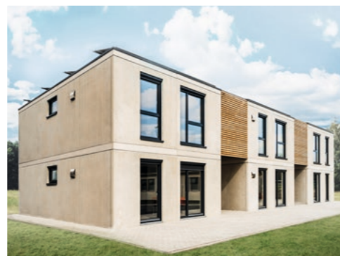
Modular construction of social housing in Schöppingen
