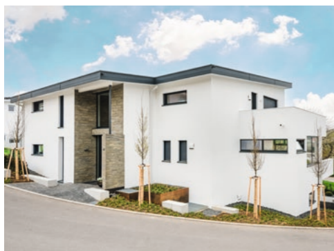
Detached house with smart home technology
