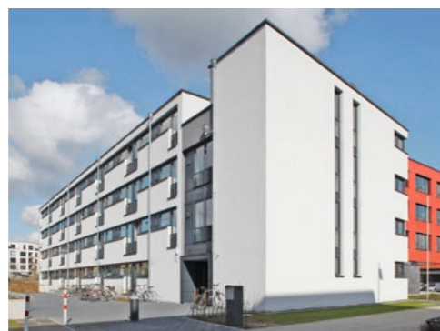
Hall of residence on Riedberg campus
