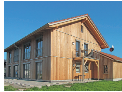
Semi-detached house in timber construction
