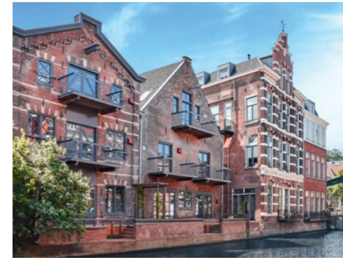
Hotel Pakasa in Leiden, refurbishment of a listed building
